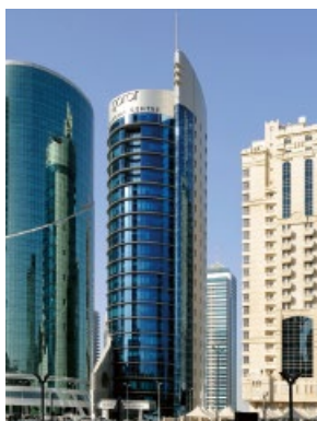
Doha, Qatar Financial Centre
